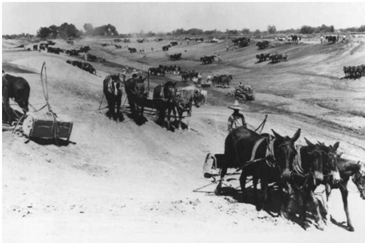
Construction of the All-American Canal
