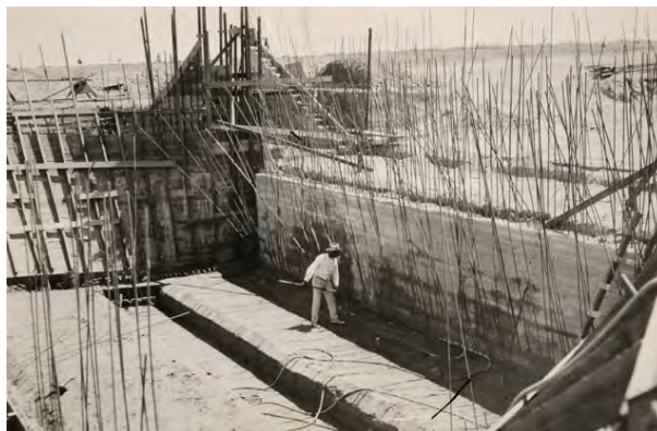
Imperial Canal Construction, 1910
