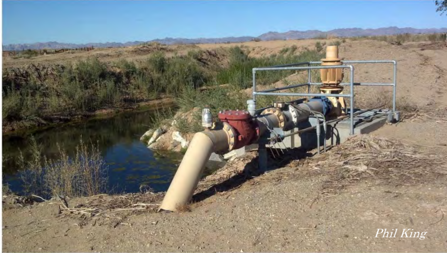
Pump in drain returning seepage to main canal (East Highline Main)
