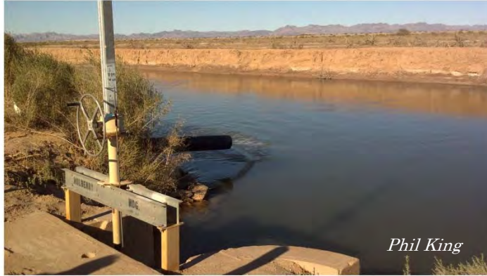
Seepage return into East Highline Main Canal
